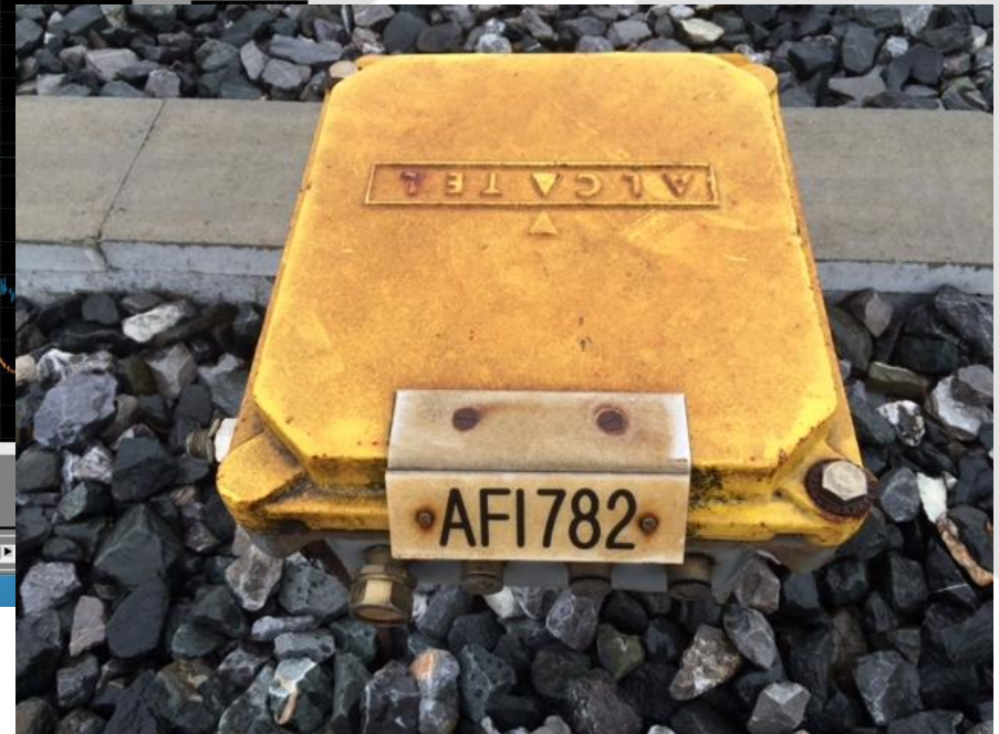
Traffic monitoring induction loop
